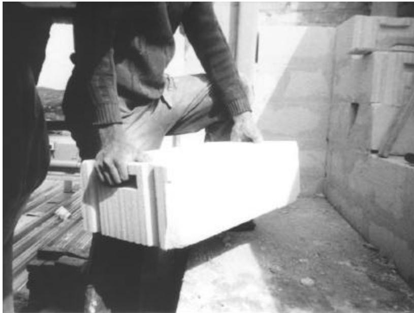
**Figure 5.** Method of handling porous silicate blocks.
