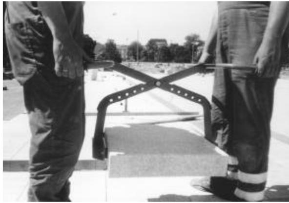
**Figure 1.** The handling of a granite tile with a mechanical lifting device.
