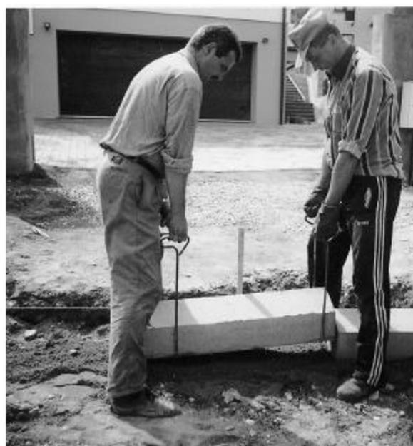
**Figure 3.** Handling the road kerb with old-type hooks.
