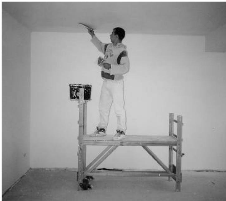
**Figure 7a.** An ergonomic bench used in puttying process.
