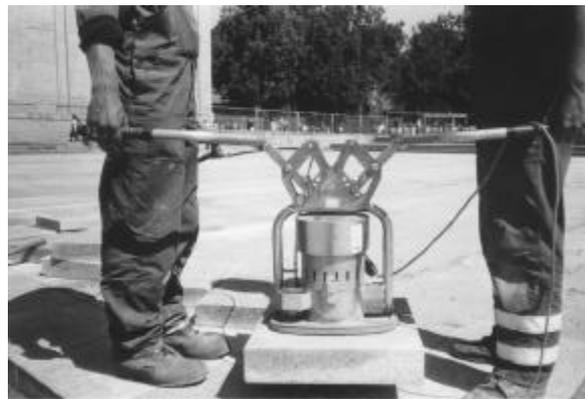
**Figure 2.** The handling of a granite tile with pneumatic lifting device.
