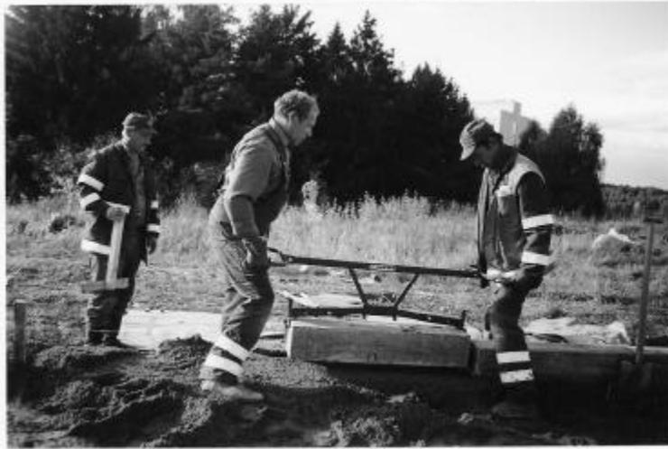
**Figure 4.** Handling the road kerb with a mechanical ergonomic device.
