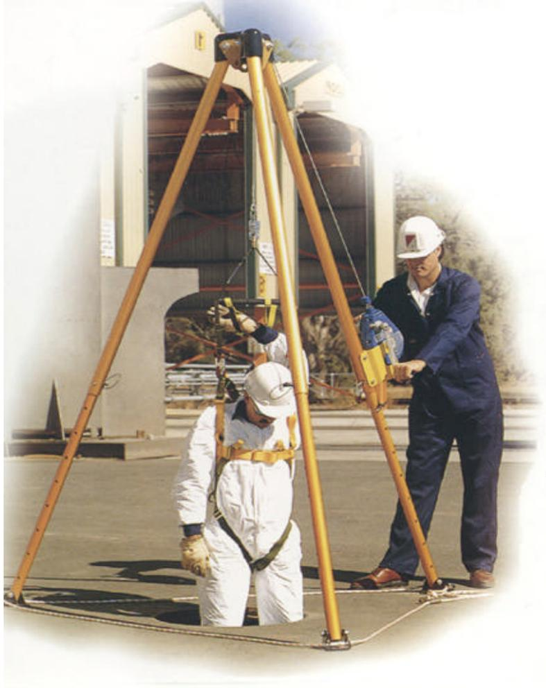
Figure 4: Height safety equipment in use during a pit entry
