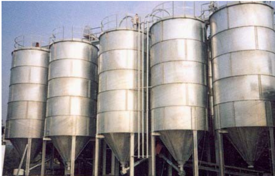
Photo 1. Examples of silos
